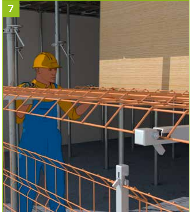
- Make sure that the mesh is in position in the slots at the top and base of the posts.
