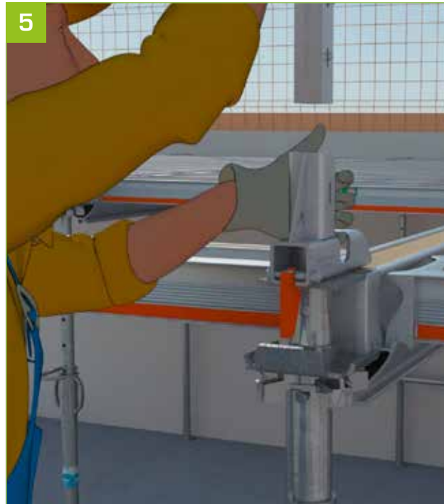
- Fit the AlphiSafe post in the adapter.
