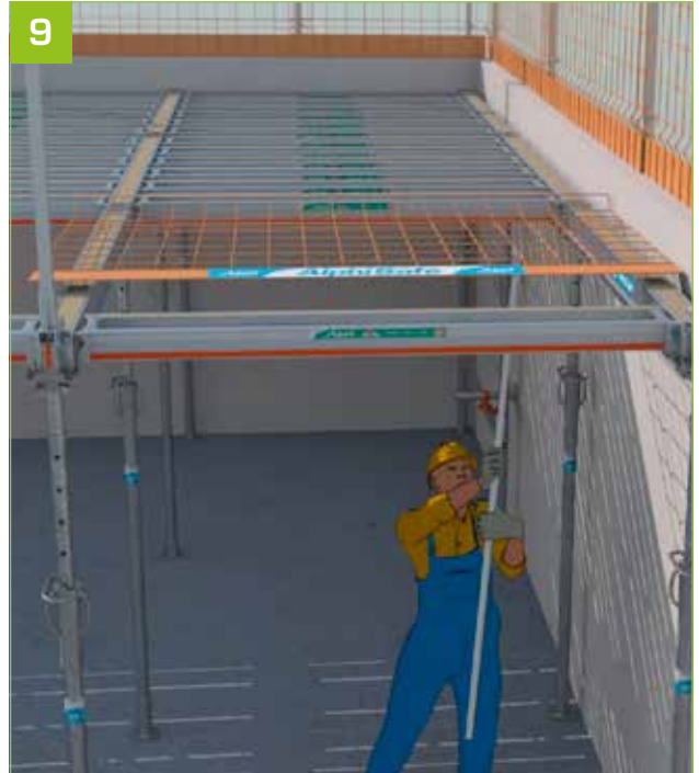
- This procedure is facilitated by using the AlphaSafe pole.
