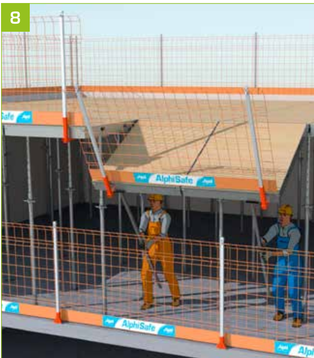
- Lift the panels using the MaxiDalle poles.
