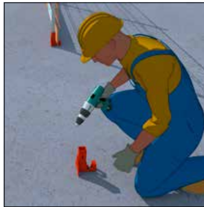
- Secure the adapter to its support. A concrete screw of at least 12 mm in diameter is recommended.
