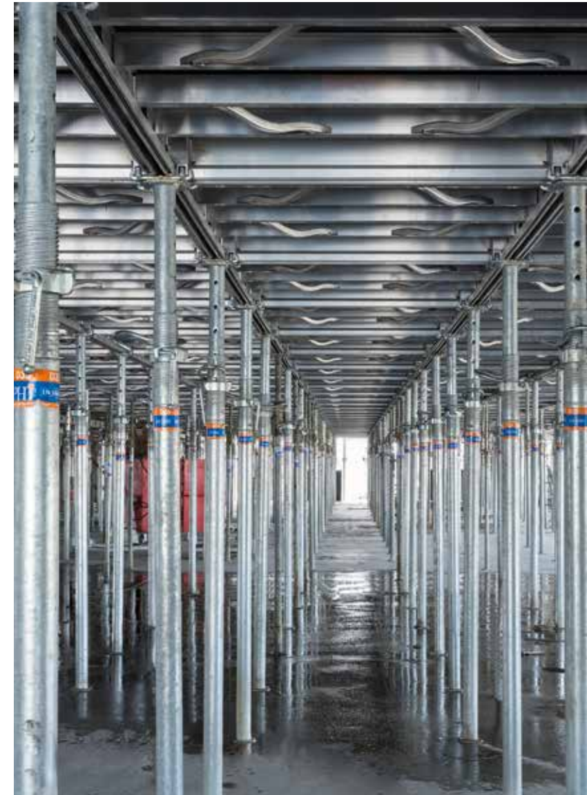
MaxiDalle formwork is particularly suitable for commercial structures
