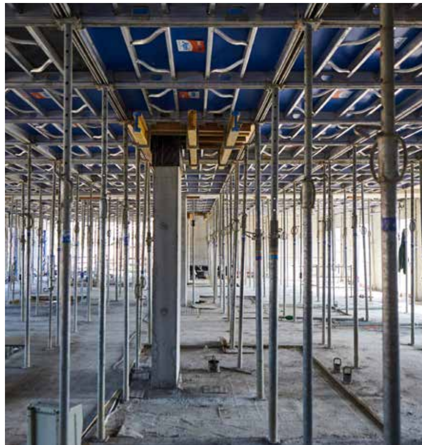
A single system, MaxiDalle, for both the floors and the overhangs
