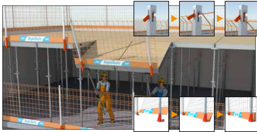
The grid is locked at the top by the anti-lifting pin and locked in rotation at the base.
