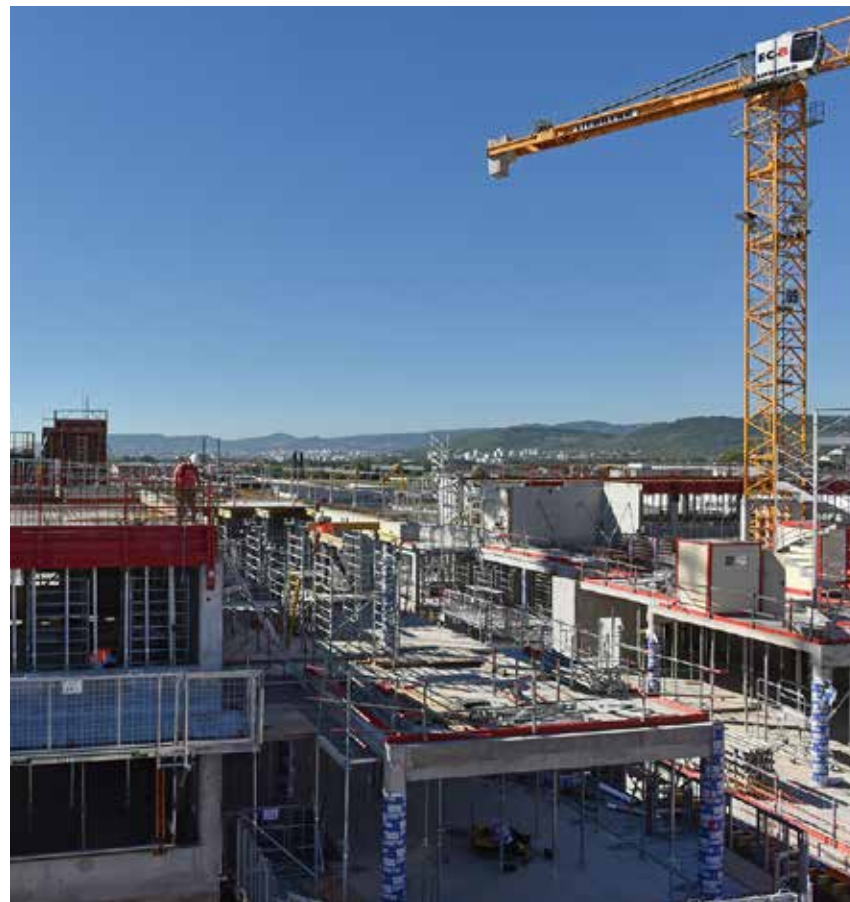
Alphi worked on all of the cast-in-place floors
