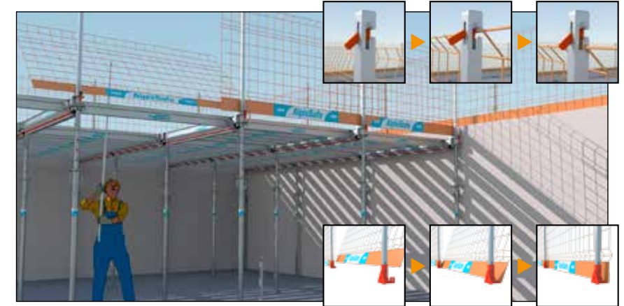
The grid is locked at the top by the anti-lifting pin and locked in rotation at the base.
