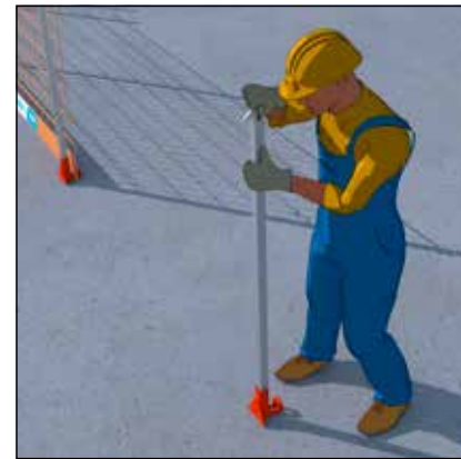
- Clip the post in the adapter.
