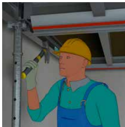
The integrated drop-head for fast removal enables a quicker turnaround of the aluminium structure.
