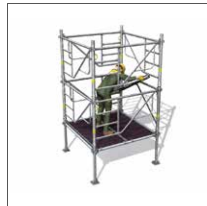
- Assemble one floor level in temporary position. - Install a 1 st 1-m plank with trapdoor.
