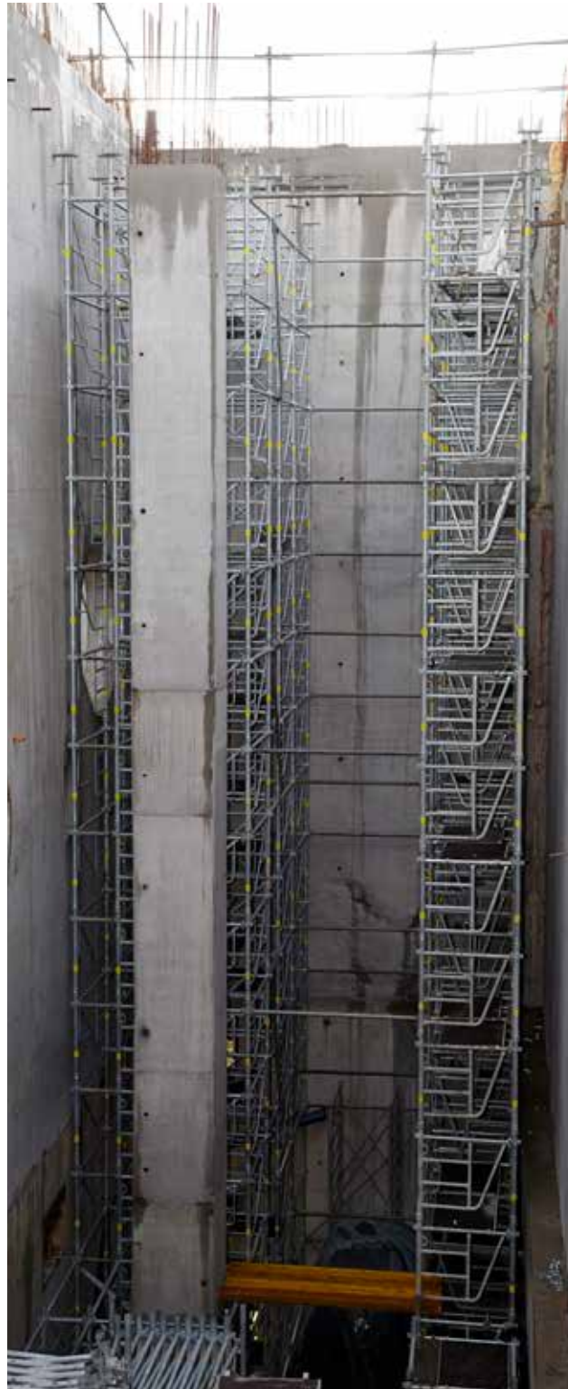
1,100 tonnes of shoring, up to a height of 49 m
