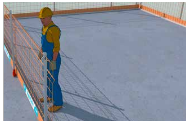
- The grid is locked at the top by the anti-lifting pin and is locked at the base.
