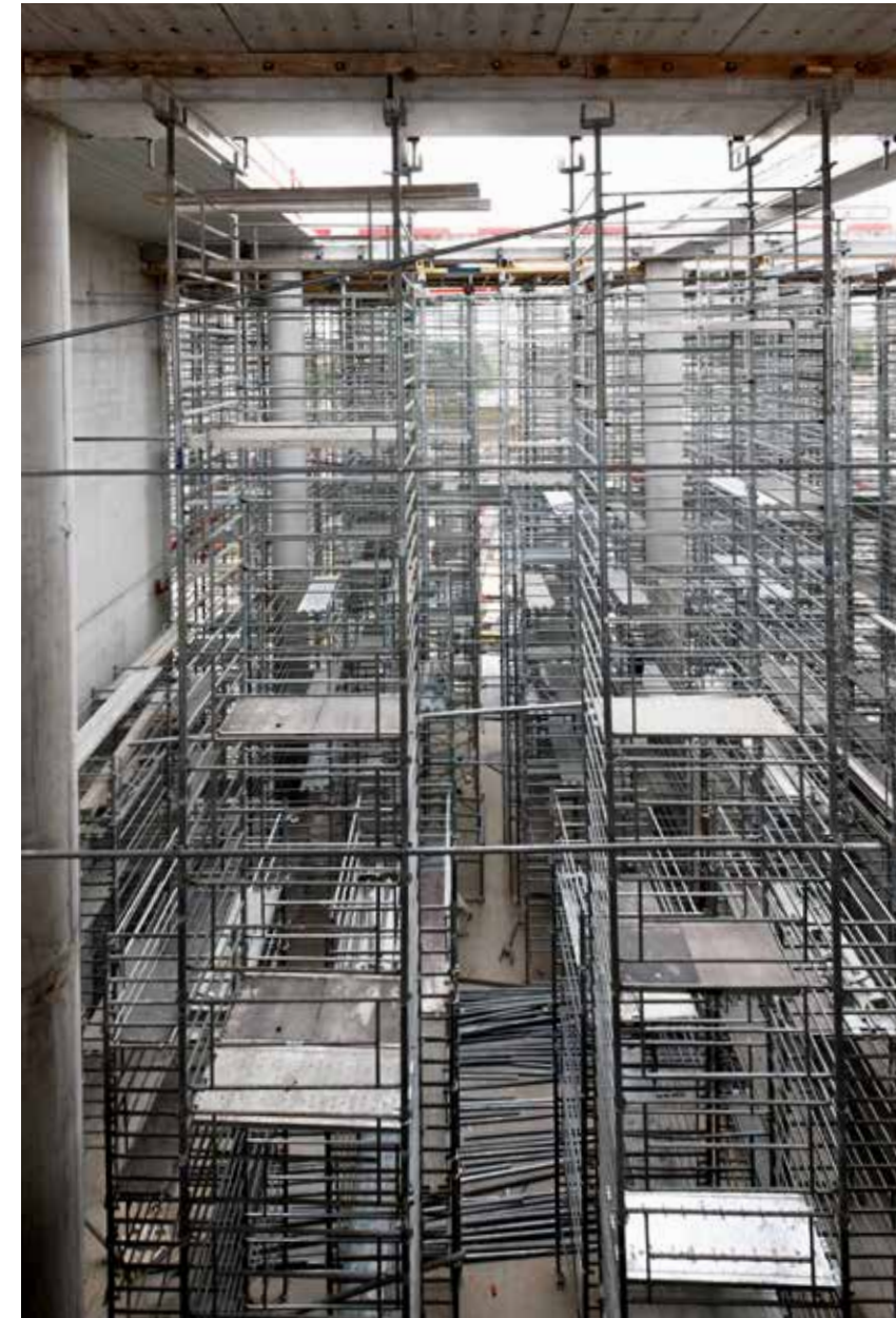
Shoring up to a height of 16 m
