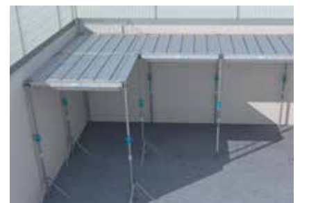
The extendable beams let you go near the cell edges
